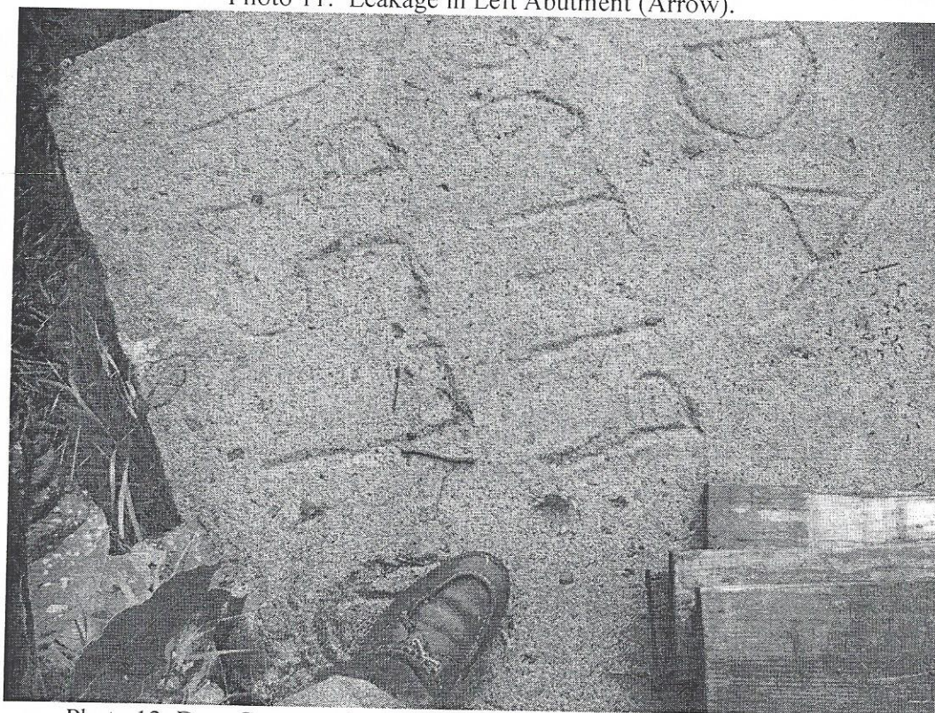
Photo 12. Dam Construction Date Imprint on Top of Left Abutment Wall.
